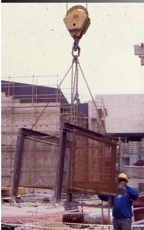
**Lowering of brick page over pallet for hoisting to the required floor level,
